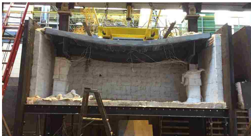
Figure 71 – Unprotected Beam after Failure
